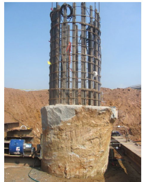
O-Cell axial shaft set up for subsequent lateral testing
