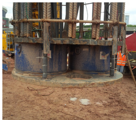
O-Cell assembly at tip of reinforcing cage
