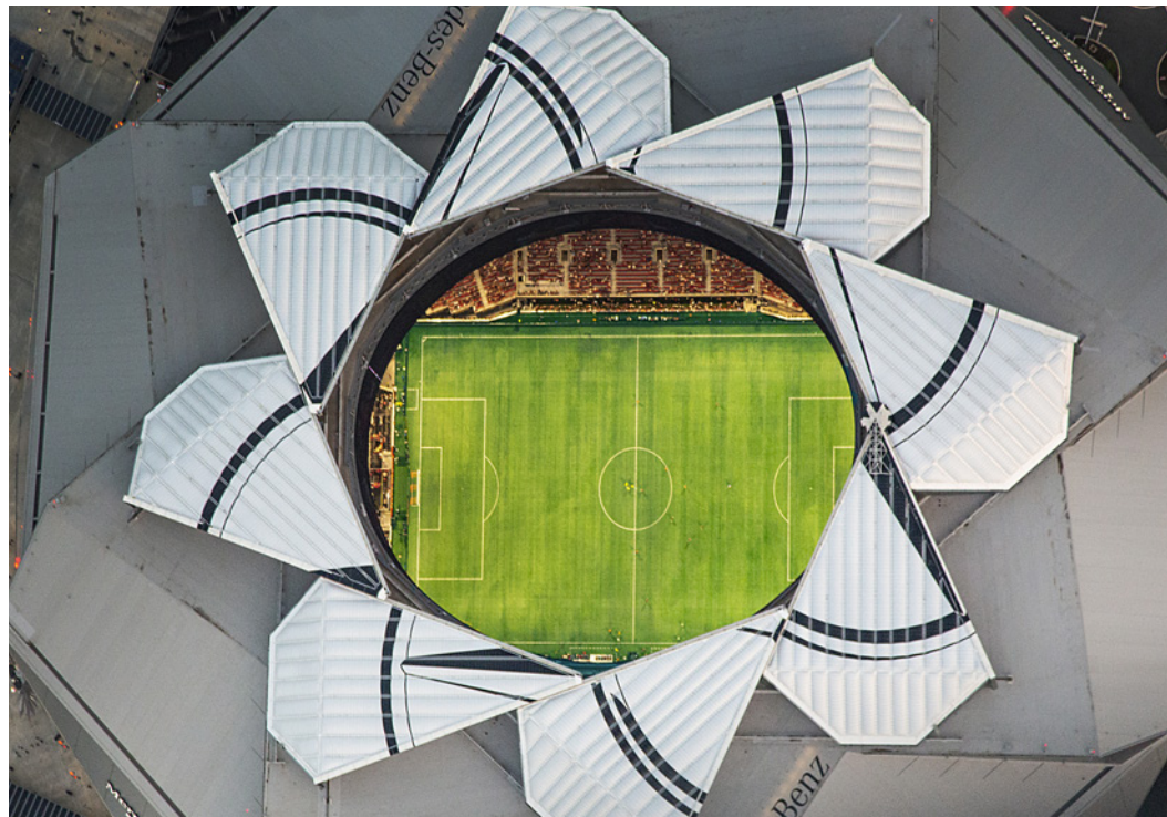
Aerial view of the stadium's retractible roof
